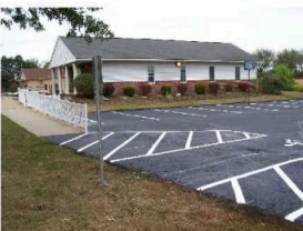
New Parking Lot
